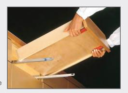
• TO ADJUST ALIGNMENT on the **Standard** wood drawers (A), slide white adjustment tab forward or backward to raise or lower the drawer box. On **Heritage** drawers (B), slide gray adjustment tab to make this adjustment. This movement will adjust the horizontal reveal on the drawer faces. For additional adjustment, loosen the screws that attach the drawer face to the drawer box and adjust.
